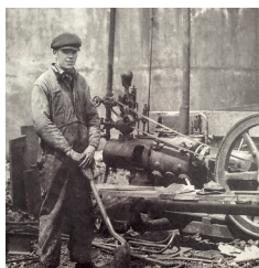
(Top) Workers inspecting the cables of the Walt Whitman Bridge during construction circa 1960. (Bottom left) In 1927, Eugene Mark Reardon operated this steam-driven pug mill, used to make blacktop. Local 825 was only seven years old. A strong labor advocate, Eugene went on to become president of Local 825, serving in the 1950s up to his retirement in 1959. (Bottom middle) Joe Steelman at a construction project site in South Jersey. (Bottom right) Richard Laveve on a job in Union County.
